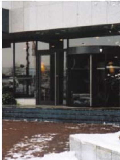
Snow and ice prevention at building entrance
