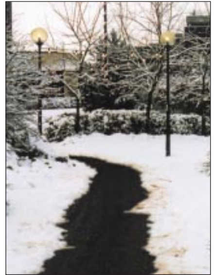
Snow and ice prevention of pedestrian walkway
